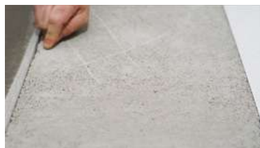
CEMENT-BASED SCREED checking hardness and cleanliness
