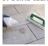
When the grout has hardened (after at least 7 days), any residue and streaks can be removed using **Fuga-Shock Eco**.
