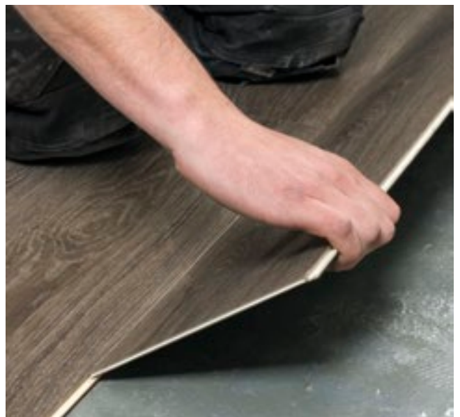
Palio Rigid 2G™ click-locking angled installation
